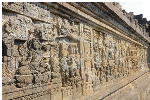
Fig. 7 The condition of the reliefs in Borobudur Temple
