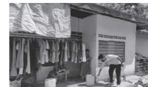
Figure 20 Architect Graduate Mr. Azam Malek from Taylors University here conducting a site assessment with one of the families affected by flood documenting the flood level and damage on the property & the livelihood of the residence
