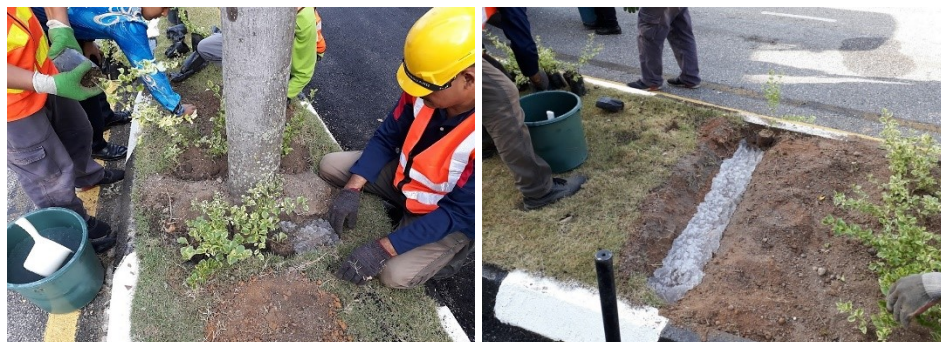
Figure 2: SAP- industrial-grade water retention material for new planting Source: Author, 2021
