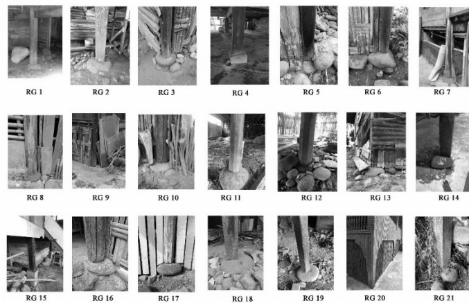
Figure 9: Elements of the Foundation Source: Desy Aryanti, 2021
