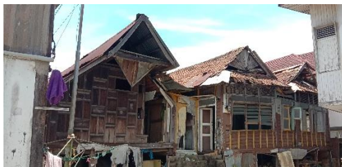
Figure 5.0: The Pemeleh in abandoned Rumah Tiang Dua Belas Kelantan (Source: Abdullah, 2021)
