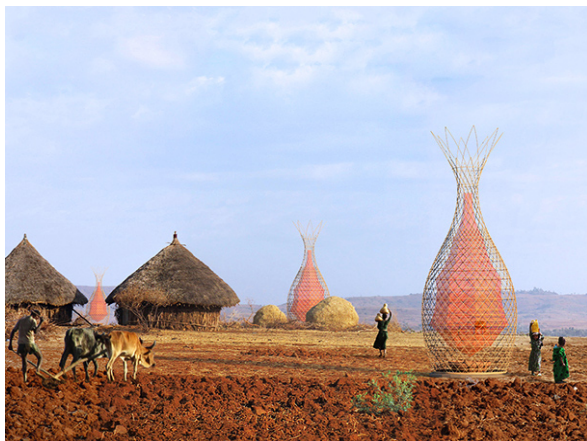
Figure 6. WarkaWater Towers Collect Drinking Water from Thin Air in Ethiopia. Source: https://media.wired.com/photos/593295e358b0d64bb35d2cf2/master/w_1600%2Cc_limit/warka6.jpg
