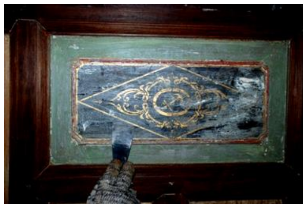
Figure 2: Mural painting made of 'air emas' discovered on the wooden paneled wall during paints scrapping work (source: JWN 2009)
